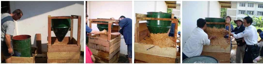
Figure 7 Fuel feeder assembling
