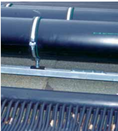
Figure 15: Example of sliding installation of pipes with anchor clamps
