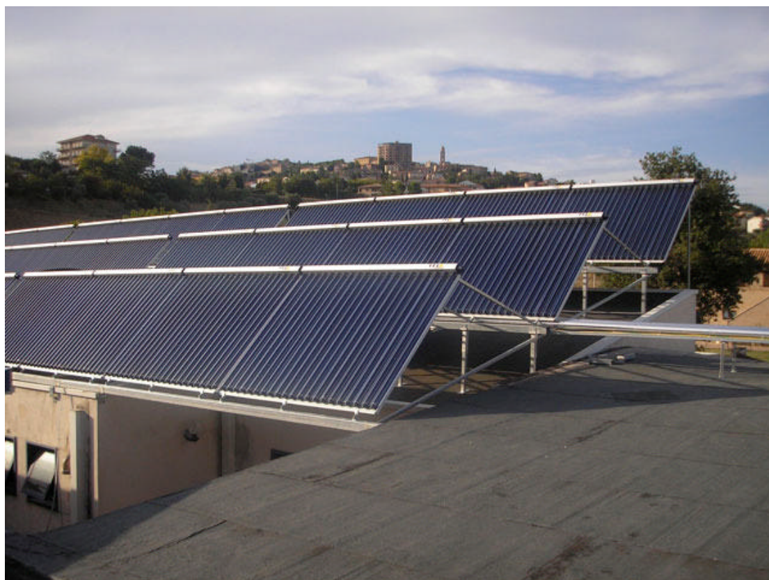
Figure 15: Swimming pool of Osimo
