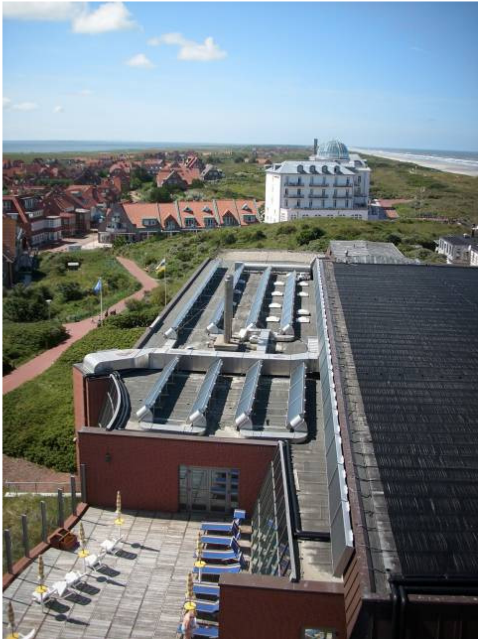
Figure 9: Combination of air collectors and unglazed absorbers
