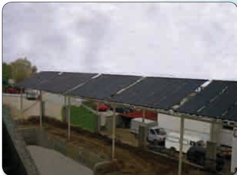
Solar polypropylene collectors for swimming pool heating, Hotel Lentzakis in Crete [Source: CRES]
