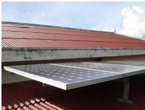
Figure 8: Installation of the PV systems for the orphan houses
