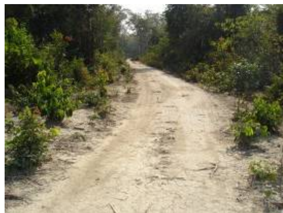
Road only can access in drying season
