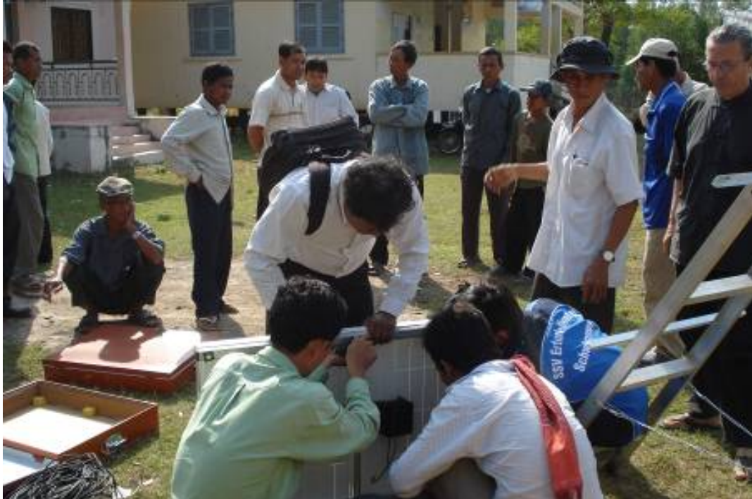
Figure 3: Installation of mobile SHS with the community members
