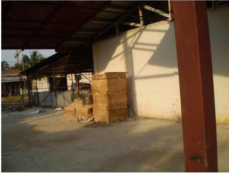
Figure 5 Location of the low cost gasifier (inside the Mechanical workshop)
