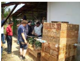
Figure 9 Gasifier is ready for test run
