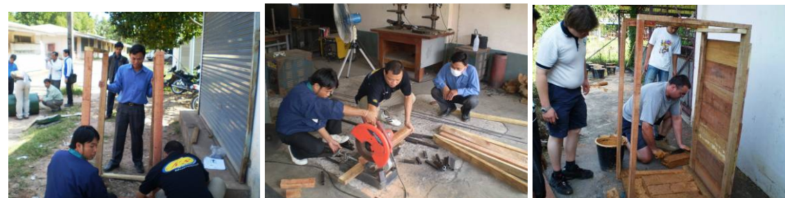
Figure 5 Wood frame construction
