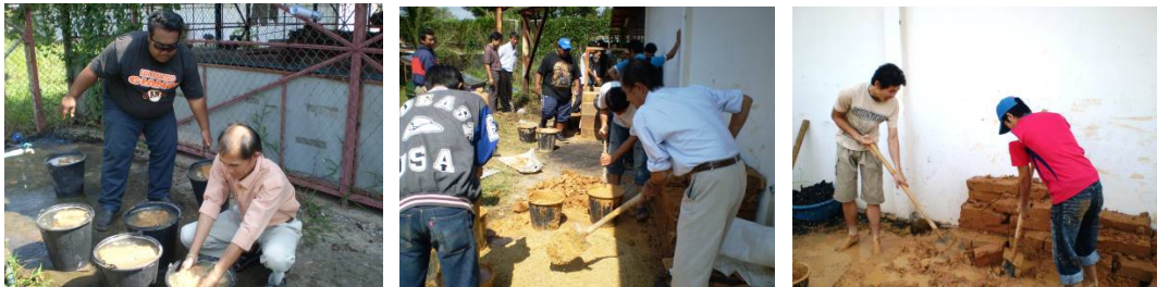
Figure 3 Groups' work: mud preparation
