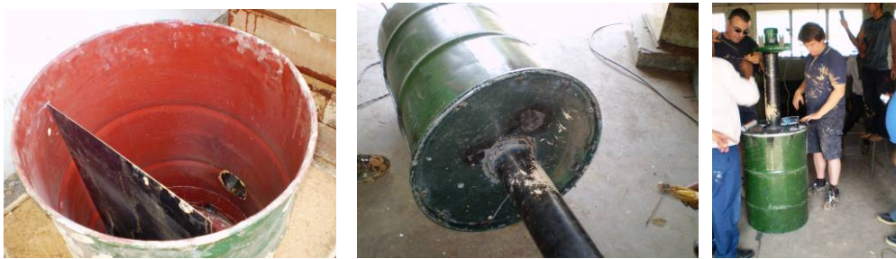
Figure 8 Ash trap and Gas Cooler assembling
