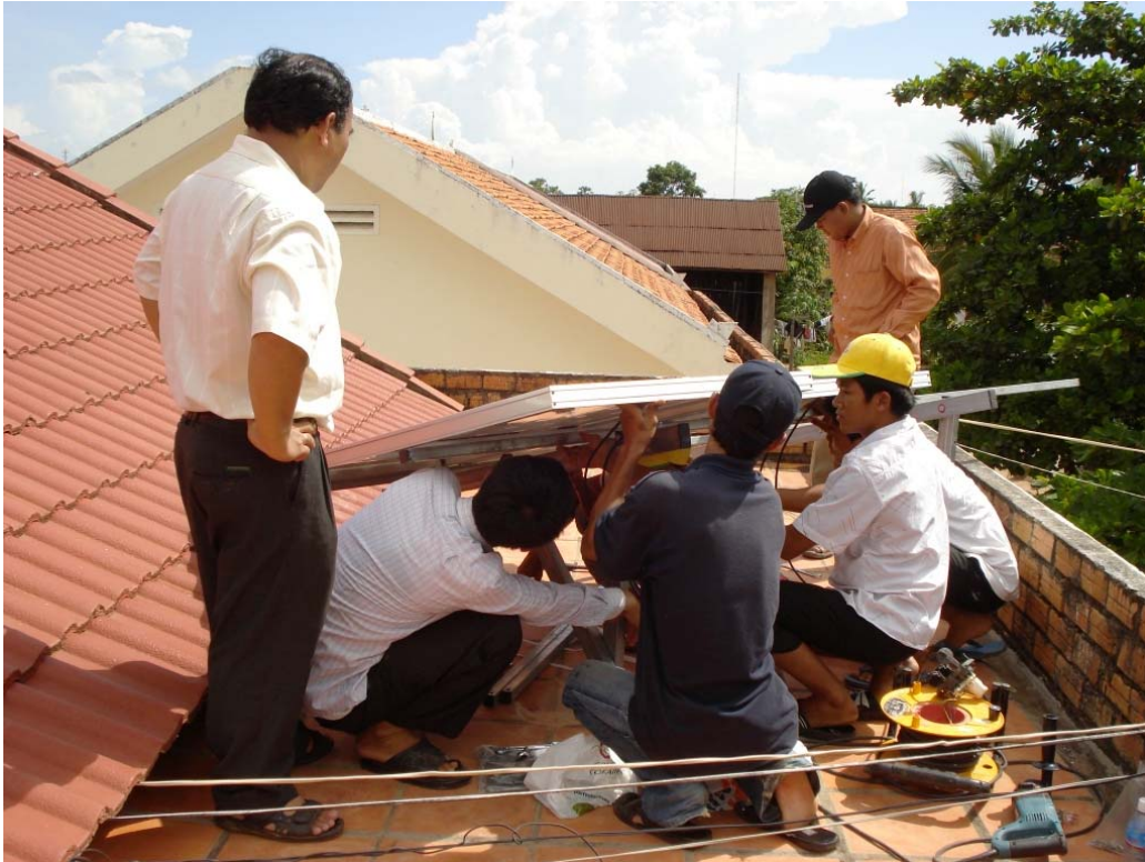
Figure 5: PV module stand installation
