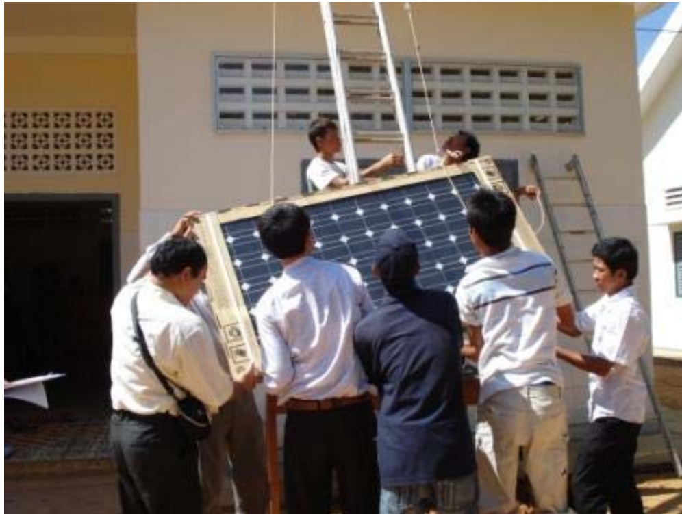
Figure 4: PV module transportation
