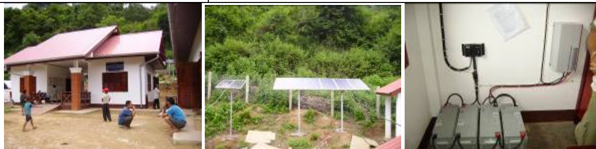
Ban Kuai health clinic and its PV system (Courtesy by Sunlabob Co.)
