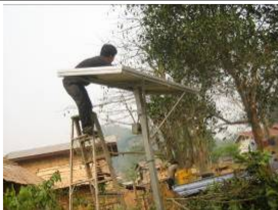
240 Wp PV array of battery charging station (Courtesy by Sunlabob Co.)
