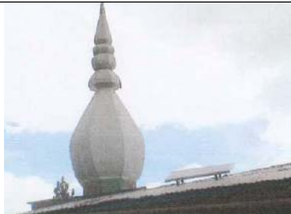
Solar module mounted on top of a mosque as part of solar home system
