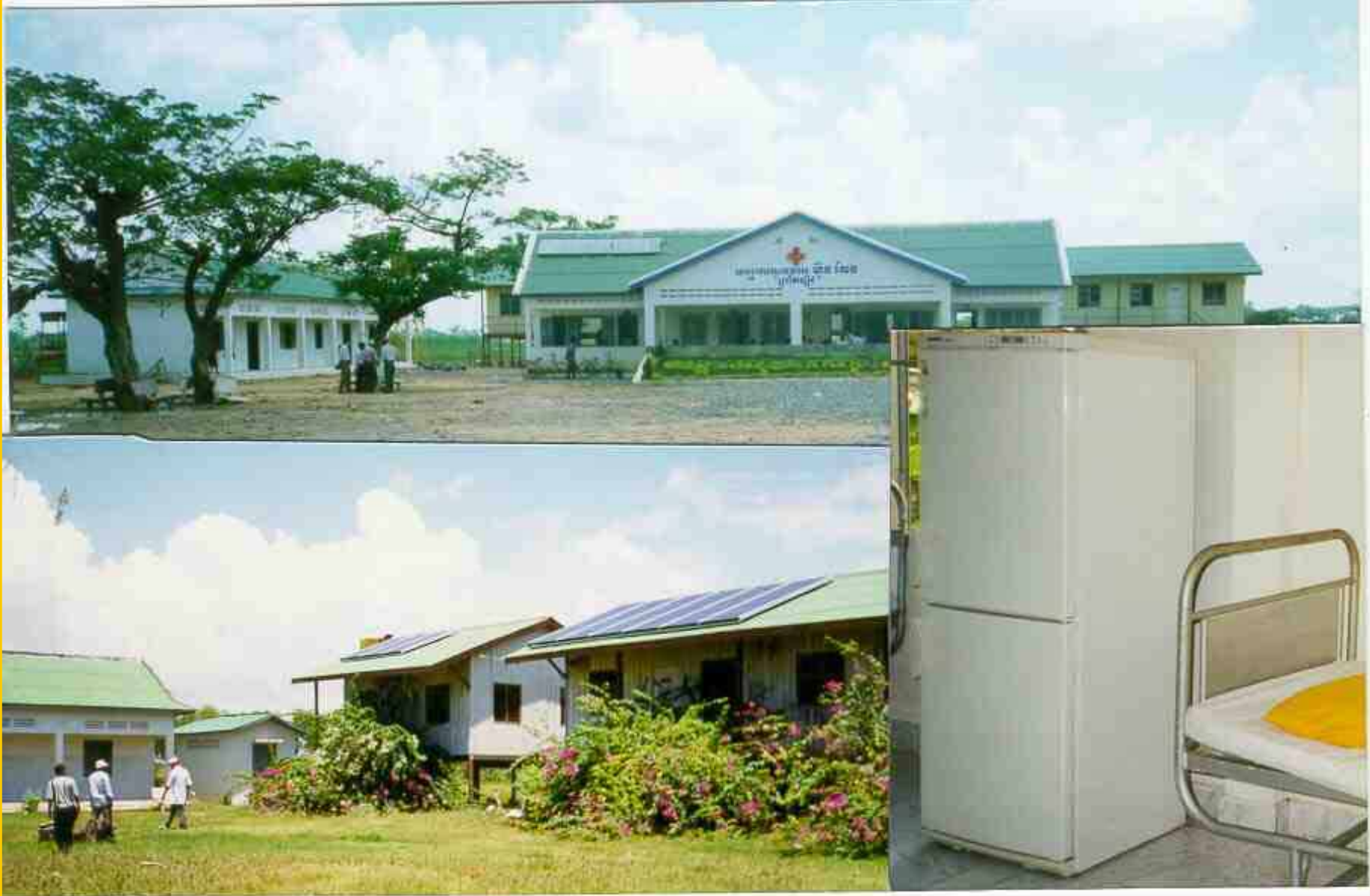
Solar System at Health Center
